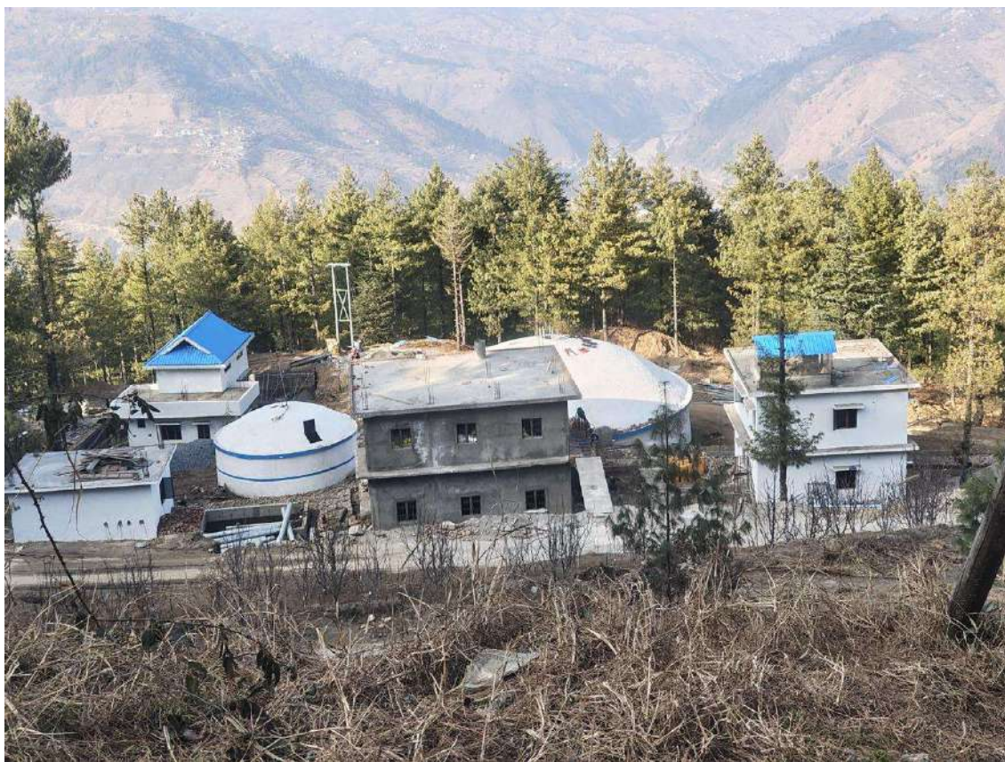
Water Storage Tank under Pabbar river Lift Water Supply Project for the Mandhol Village
